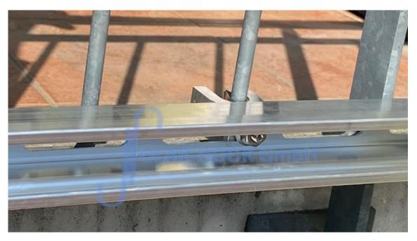
Figure 11/mounting rail and special clamp from outside
