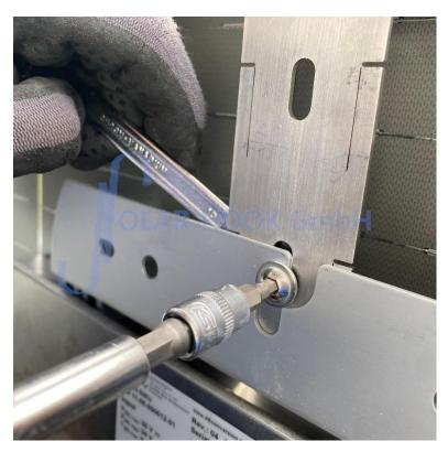
Figure 6 I screw the inverter onto the SOLAR-HOOK mounting bracket
